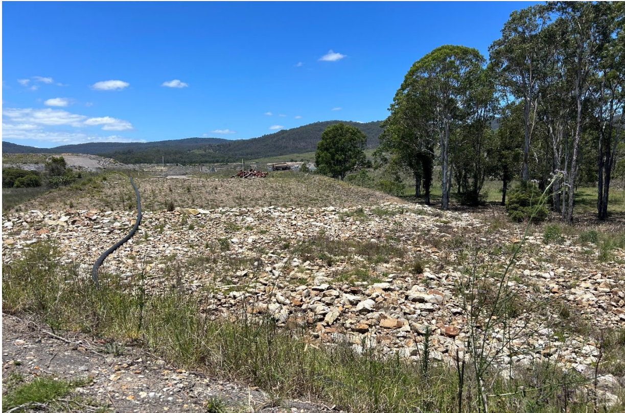
Plate 3 – Roseville Haul Road rehabilitated area with mine water transfer pipeline
