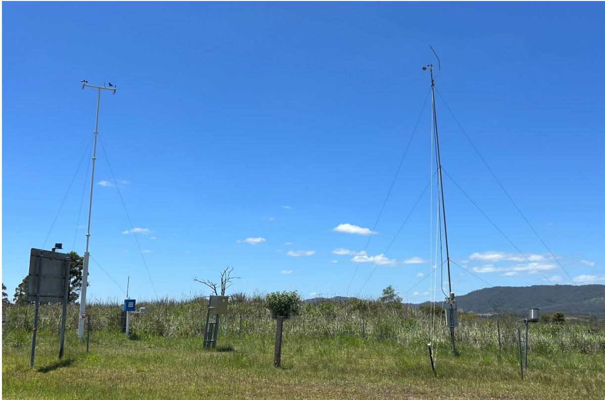
Plate 9 – Meteorological monitoring station
