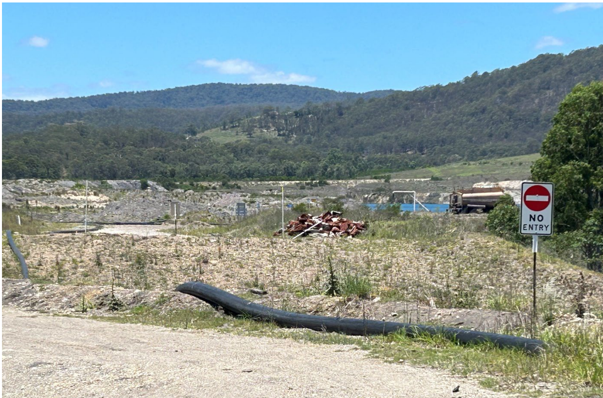
Plate 4 – Disassembled culvert atop of Roseville Haul Road and rehabilitated area
